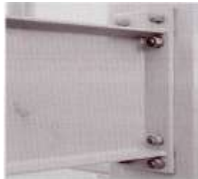
Gambar 4.6. Penghubung Kaku ( Rigid Connection )
