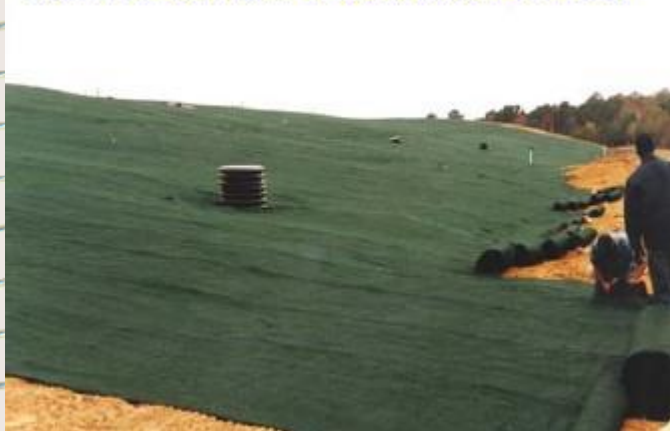
Geomat rolls used for erosion control
