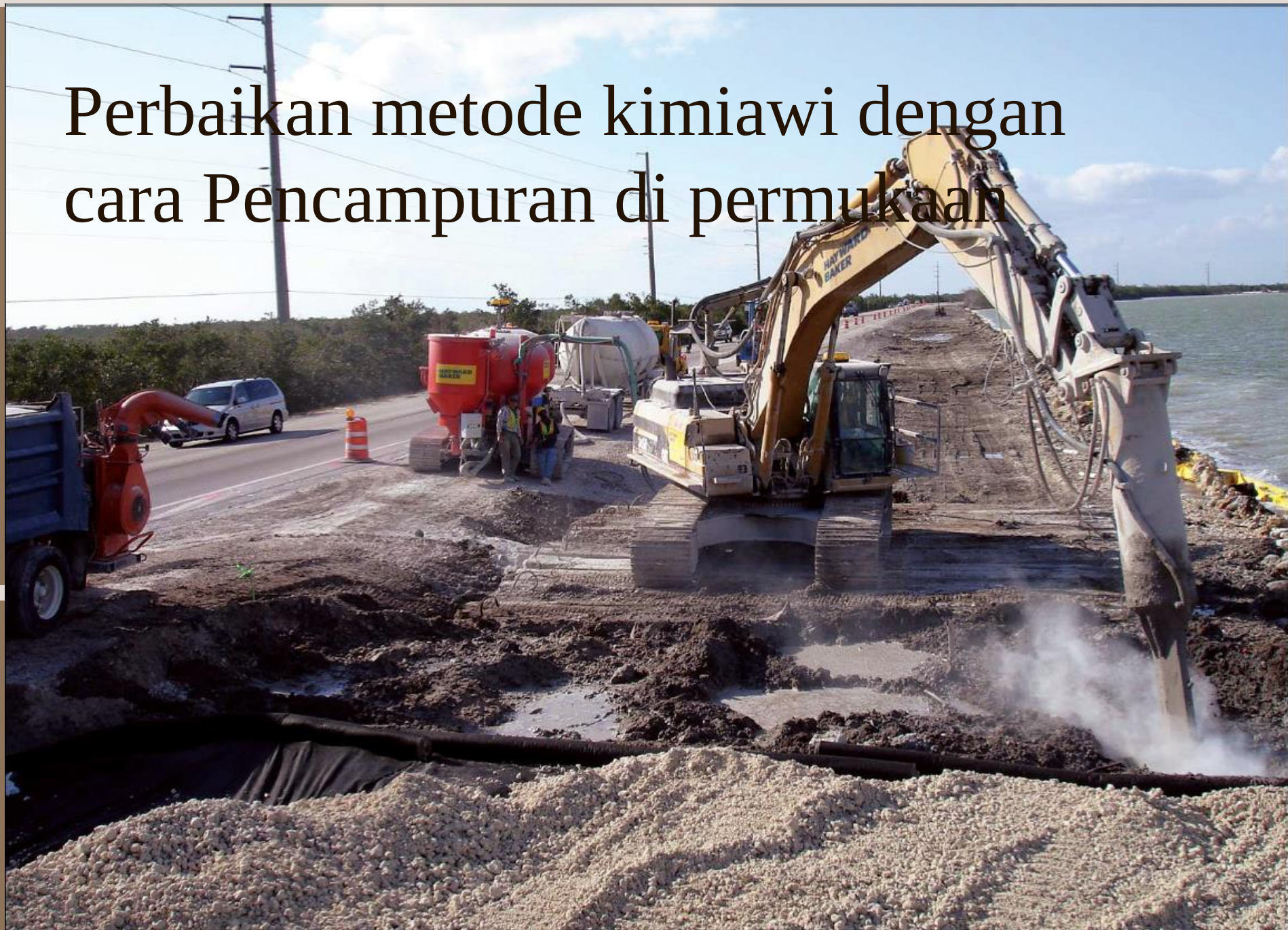
Mass dry soil mixing of soft organics for ground improvement to support a highway widening in Key Largo, Florida.
