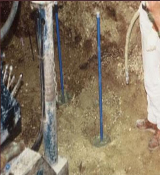
□ Compaction Grouting/Sementasi Pemadatan
