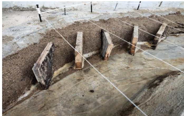
Figure 3. Placement of the 30° crib slope angle
