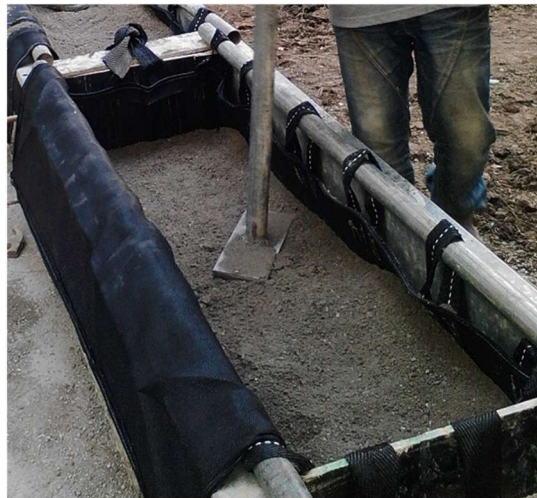
Figure 23: Filling and compaction of fine RCA/fine RAP inside geobag
