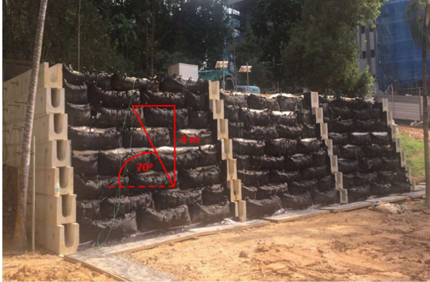
Figure 25: Completed GBS slopes at field pilot study site Orchard Boulevard
